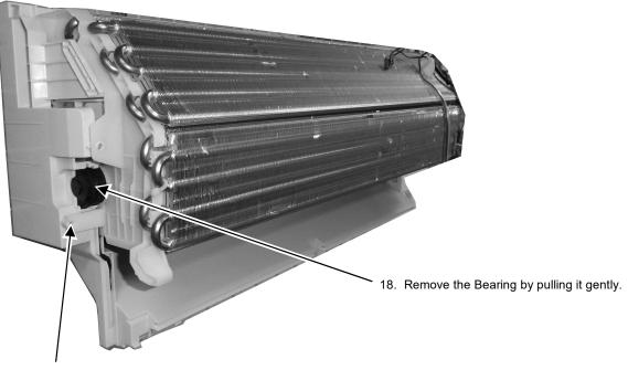
17. Remove the screw from the Evaporator.
