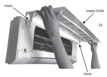
Align the intake grille hooks into the slot.
