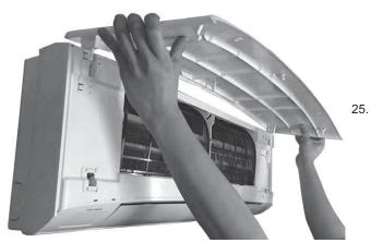
Then slightly bend the intake grille and push in the hooks into the slot.
