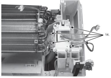
Remove the 4 screws holding the control board, then pull out the control board.
